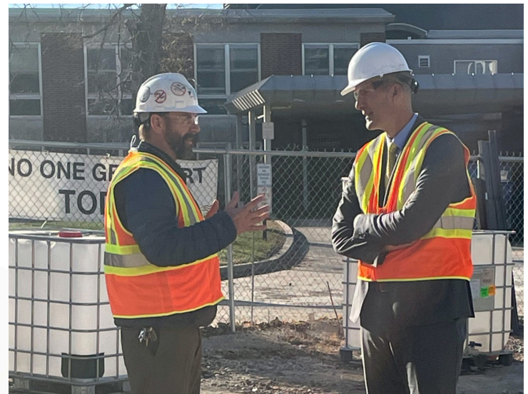
Dave Clifford, Veterans' Home at Quincy Chief Engineer, tours the construction site with Director Terry Prince.
