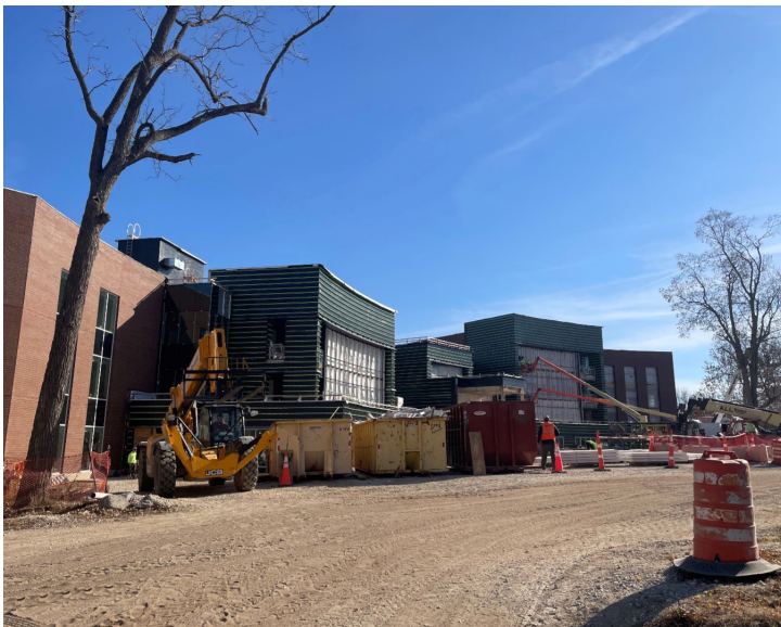
Veterans' Home at Quincy construction 75 percent completed.
