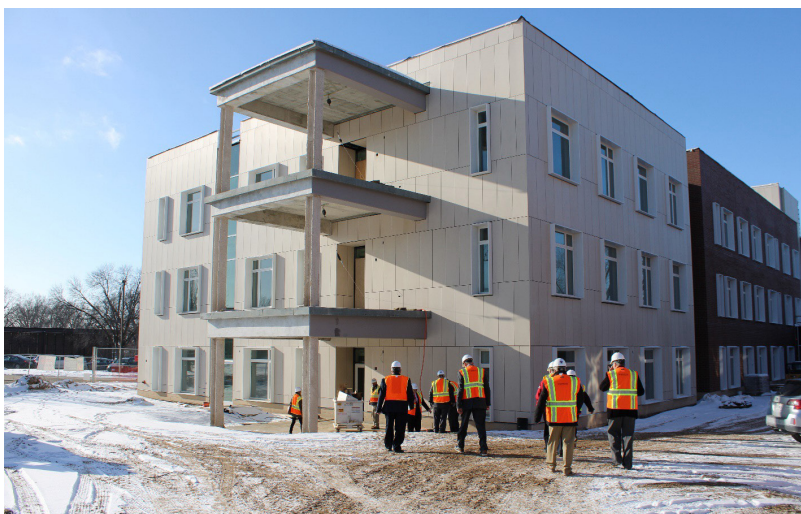
Construction of the new Veterans' Home at Quincy is underway.
