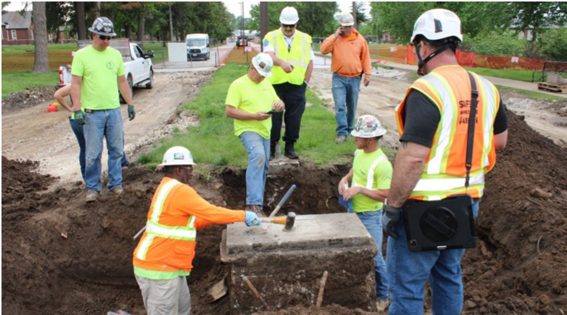
The construction crew unearths the time capsule.
